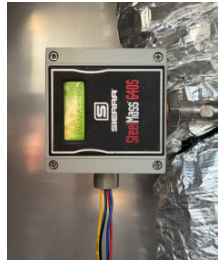
(b) insertion mass flow meter
