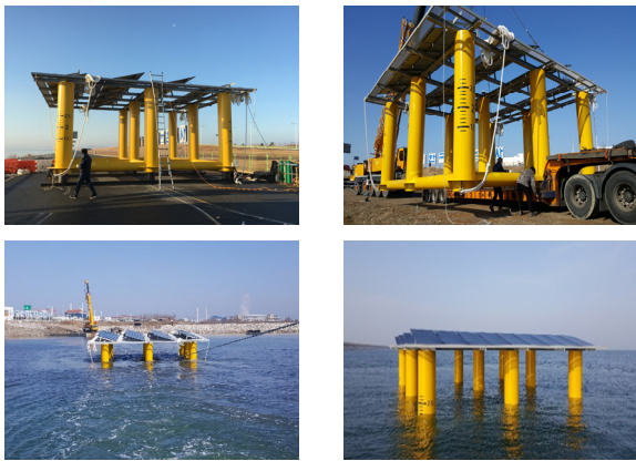
Fig. 2. Installation of offshore PV
