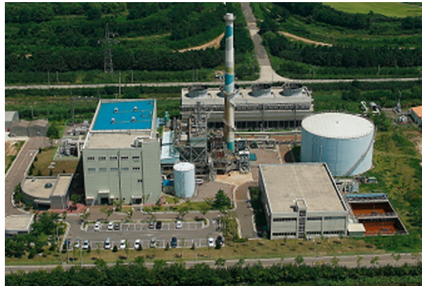
Fig. 1. 50 MW LFG power plant of S Landfill
