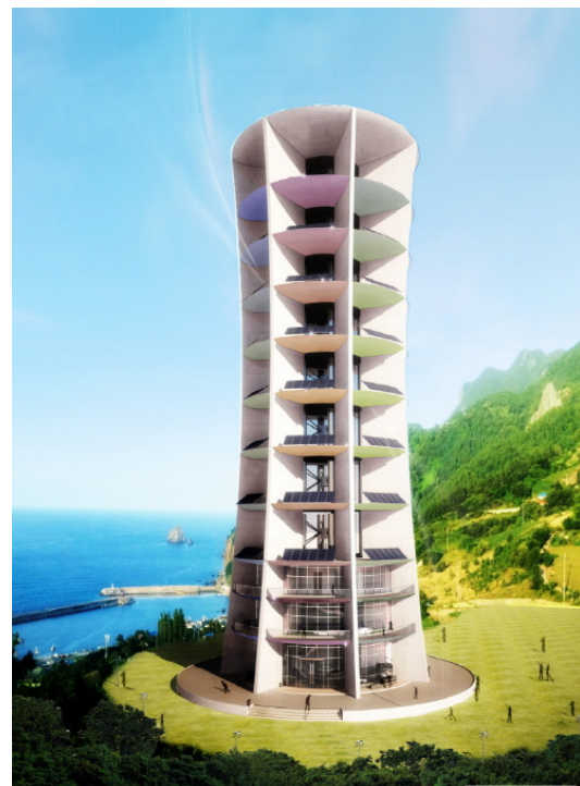
Fig. 1. View of wind power tower with VAWTs
