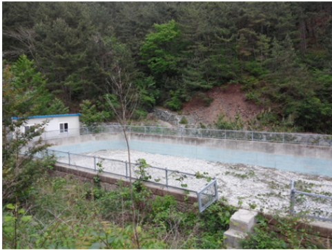
Fig. 6. View of mine water treatment facility in the Samsan Jeil mine in Korea
