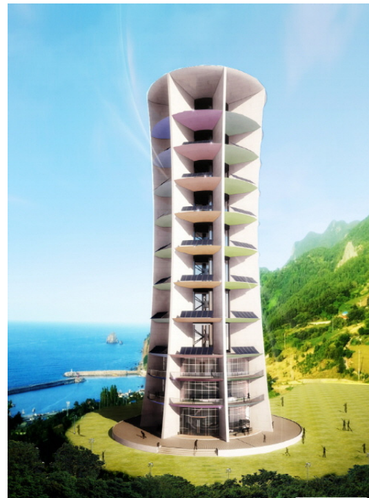
Fig. 1. View of wind power tower with VAWTs
